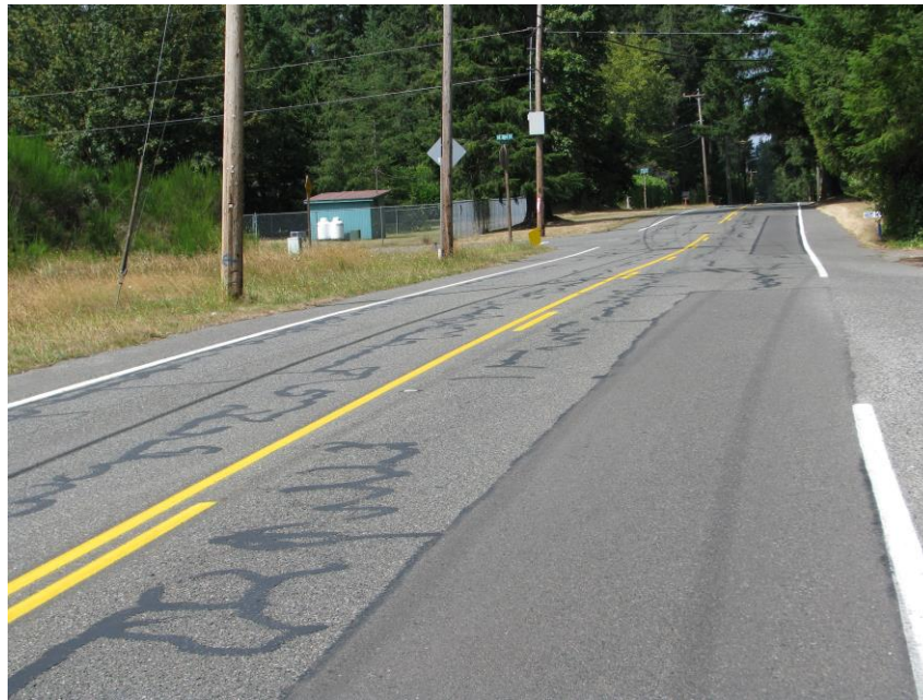
‘224 th Ave Patching and Crack Sealing Improvement in Preparation for Chip Seal’
